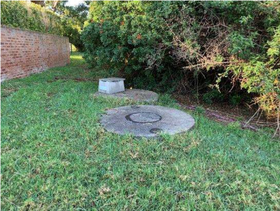
Image 6.8.1 View of septic systems observed on the site
